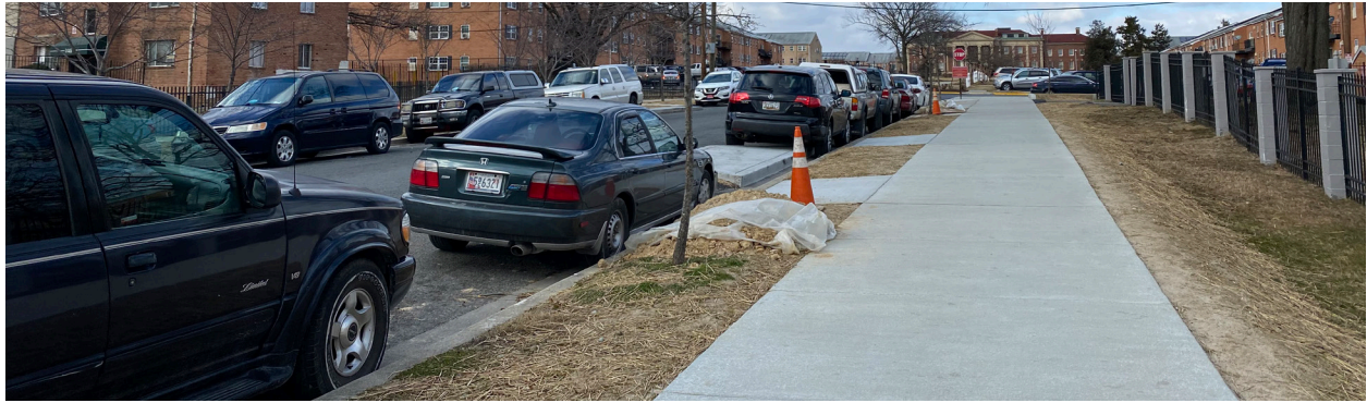
15th Avenue has an eight-foot-wide sidewalk on the east side that can function as a shared-use path.
