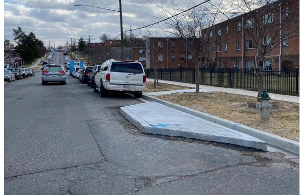
Recently installed curb extension on 15th Avenue.
