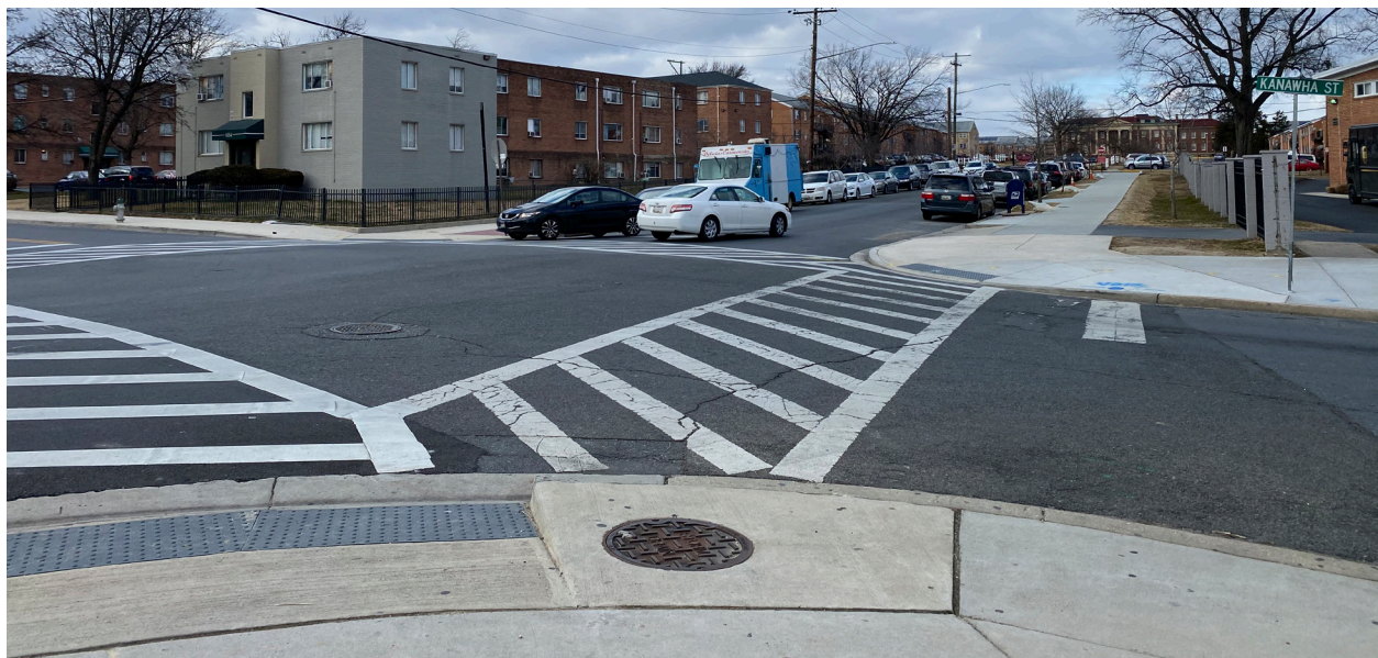
15th Avenue and Kanawha Street intersection has marked crosswalks, sidewalks, and ADA-compliant curb ramps.
