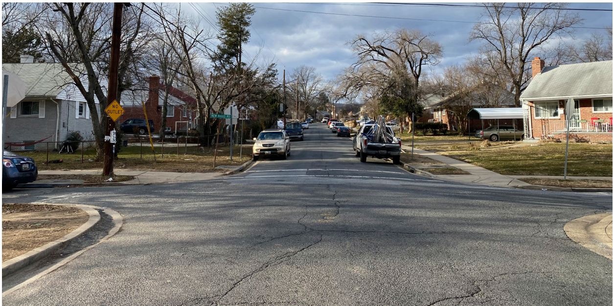
Keokee Street is 25 feet wide between curbs.
